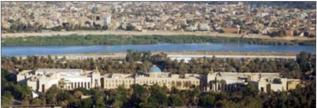
An aerial view of the Baghdad Republican Palace (where the CPA was headquartered), in the centre of the 'green zone' in Baghdad.
